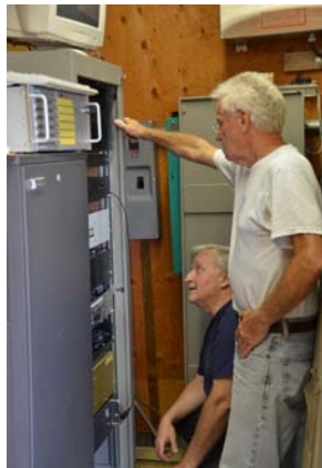
Don K9NR & Ken W9IE working on the 444.800 repeater install
