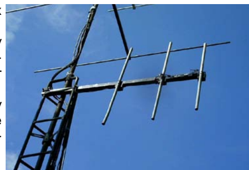
The finished antenna in position on the tower
