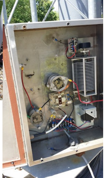
Motorized and remotely switched components inside the tuner housing
