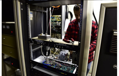
4...Bill N9OE starting installation of new controller.
